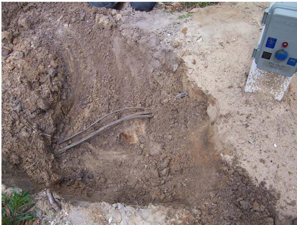
**Figure 15. Picture taken on 04/20/09 of Norweco system with wires strung across the pump tank lid preventing access. No sampling port was installed. Maintenance records indicate the effluent was visually inspected.**
