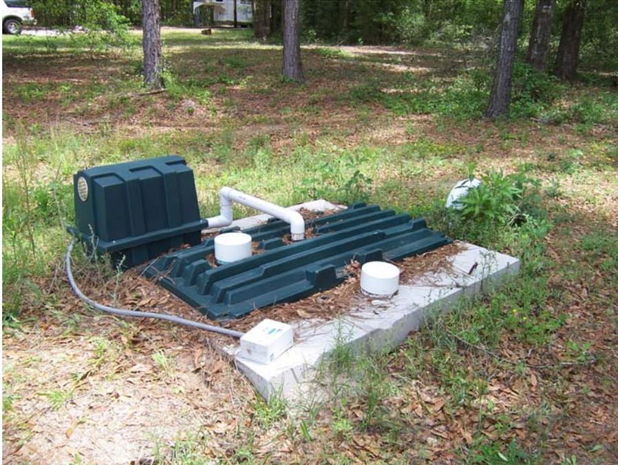
**Figure 12. Picture taken on 04/16/09 of a FAST system with the unwired control box lying on the exposed tank. The system was in use with sewage, but no electricity.**
