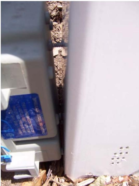
**Figure 13. Picture taken on 04/16/09 of Norweco system with the wiring to the control box not connected. There was power to the pump, but not to the aerator control box.**
